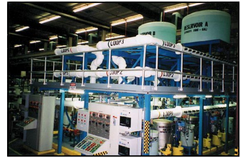
Distribution System Simulator - Front View
