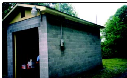
Coalwood, WV Treatment Plant Location.
